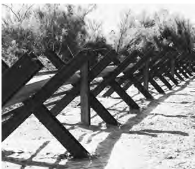
Courtesy of Border Patrol Big Bend Sector New barriers have been installed at the border to prevent illegal vehicle crossings.
