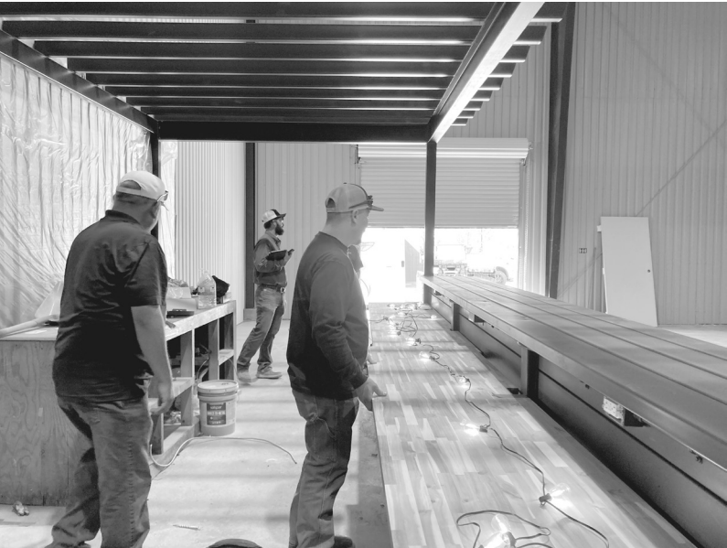
The MAC’s new serving station. Construction is expected to wrap this week.
