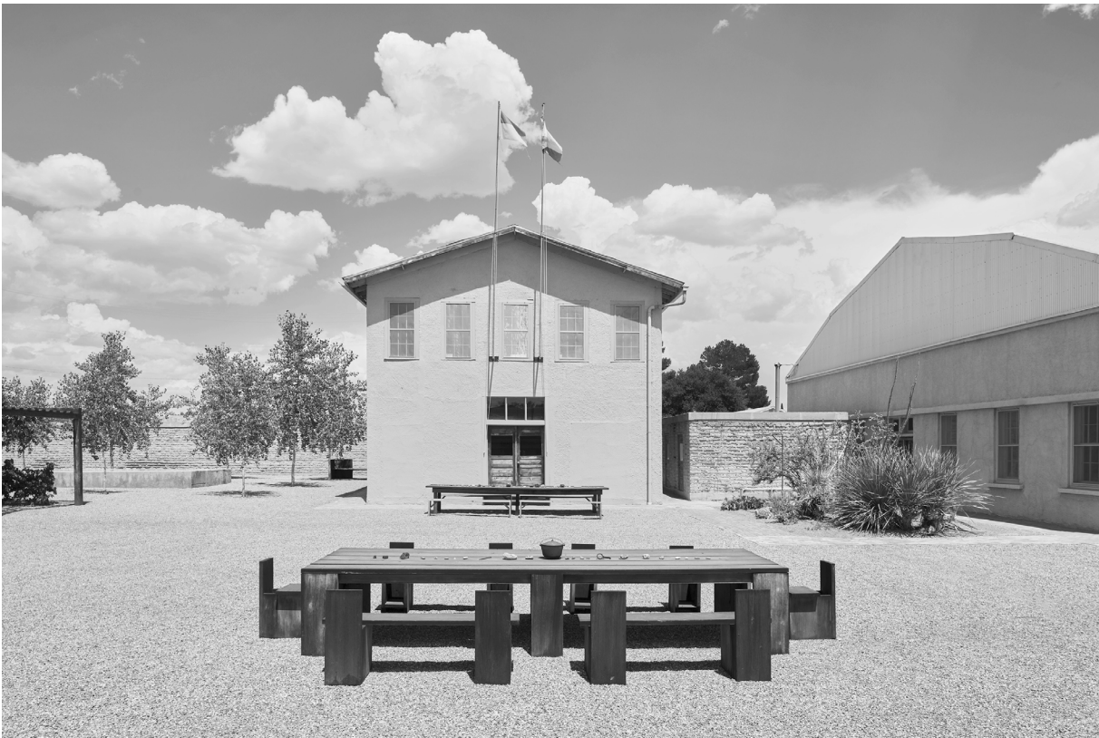
Courtyard, La Mansana de Chinati/The Block, Judd Foundation, Marfa, Texas.Photo:Alex Marks© Judd Foundation.Donald Judd Art © 2025 Judd Foundation / ArtistsRights Society (ARS), New York.Two-Story Building, La Mansana de Chinati/The Block, Judd Foundation, Marfa, Texas.Photo:Alex Marks© Judd Foundation.
