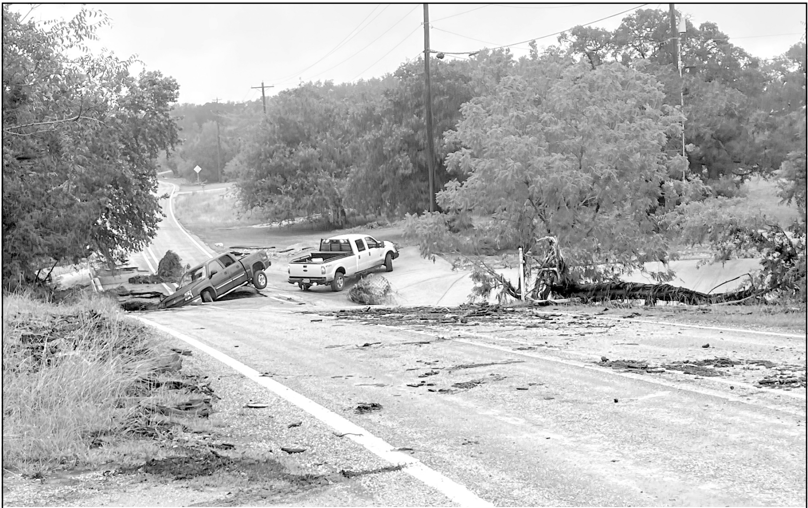
In the path of the flood Photo courtesy of Hilary Scruggs Beebe Stranded vehicles litter a low water crossing near a cabin in Hunt, Texas, owned by the family of Marfa resident Hilary Scruggs Beebe. Beebe and her family narrowly escaped the historic flood that ravaged Kerr County on the morning of July 4, claiming the lives of over a hundred people and counting. See page 2 for more.
