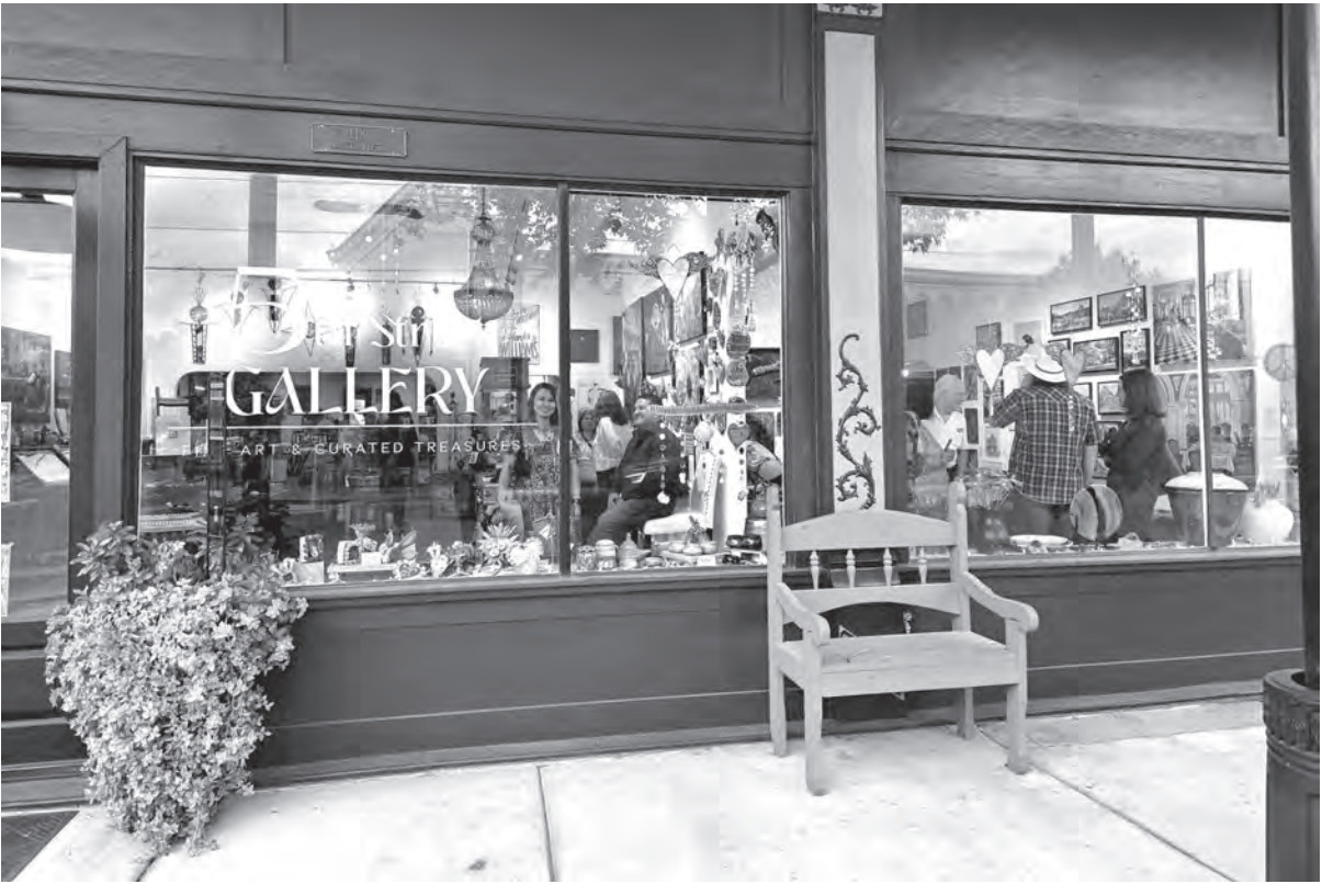
Alpine’s 5th Street Gallery resides inside the former Masonic Lodge
