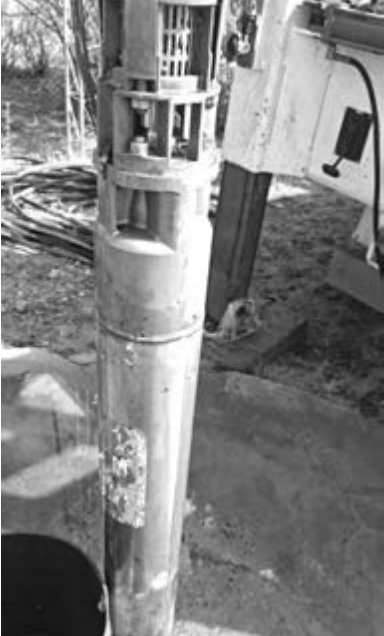
Workers examine a failed pump and discover other problems with the aging well.
